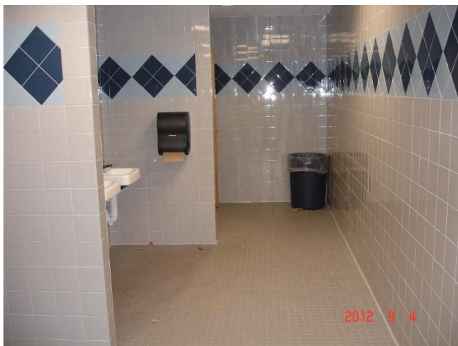
Restroom with Floor Replaced
