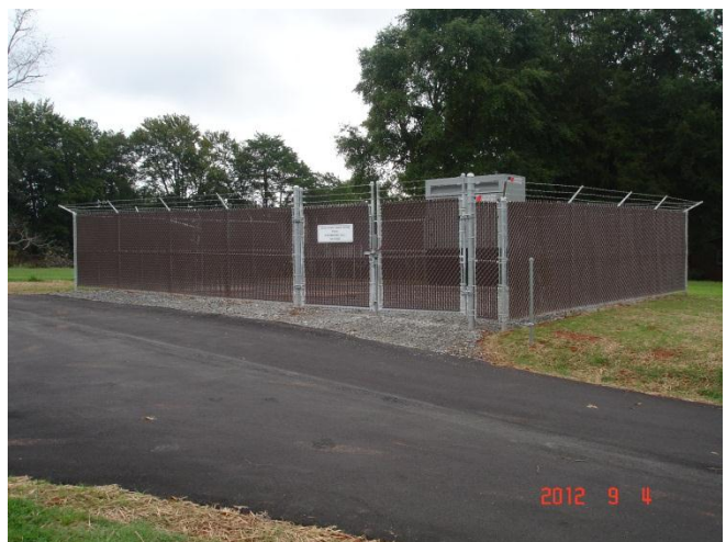
Sewer Pump Station Completed
